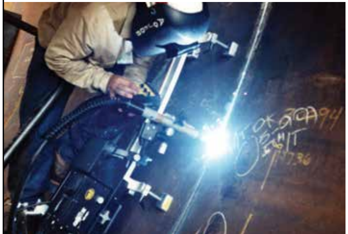
Shown Above - Vertical linear weave welding with ARM-2480 Support Bar w/ Magnets
