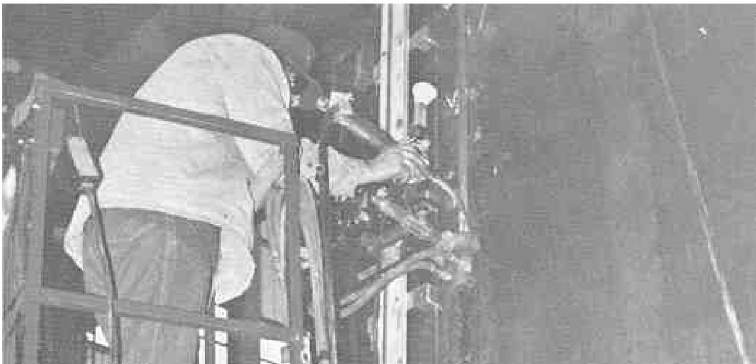
The BUG-O-VERT being used in the electroslag process.
